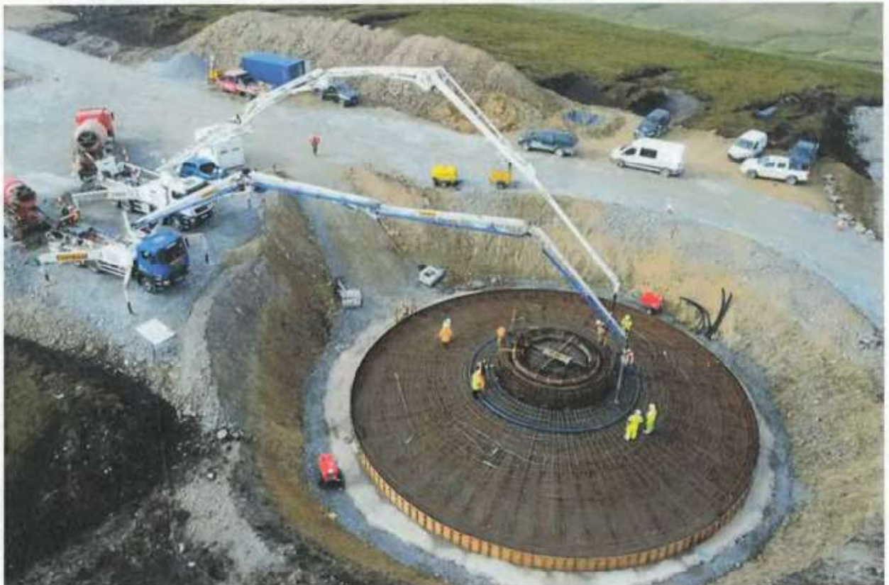
Plate 3.1: Turbine Foundation under Construction with Adjoining Crane Pad 5
