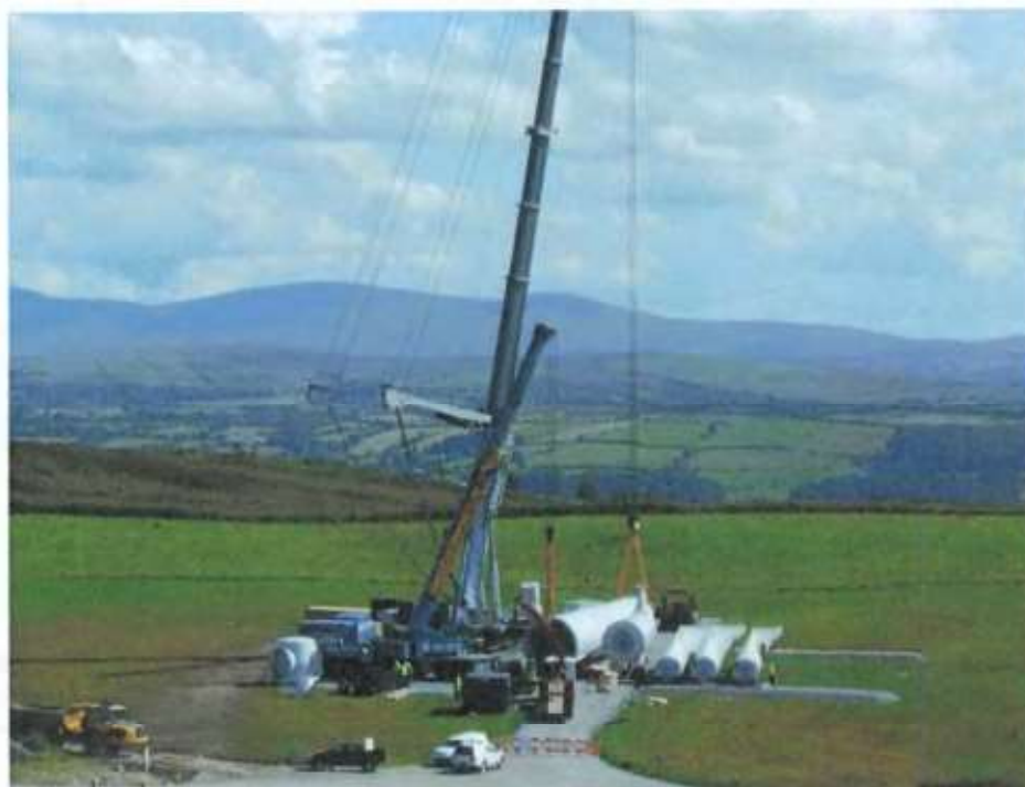
Plate 3.3: Wind Turbine Erection 7
