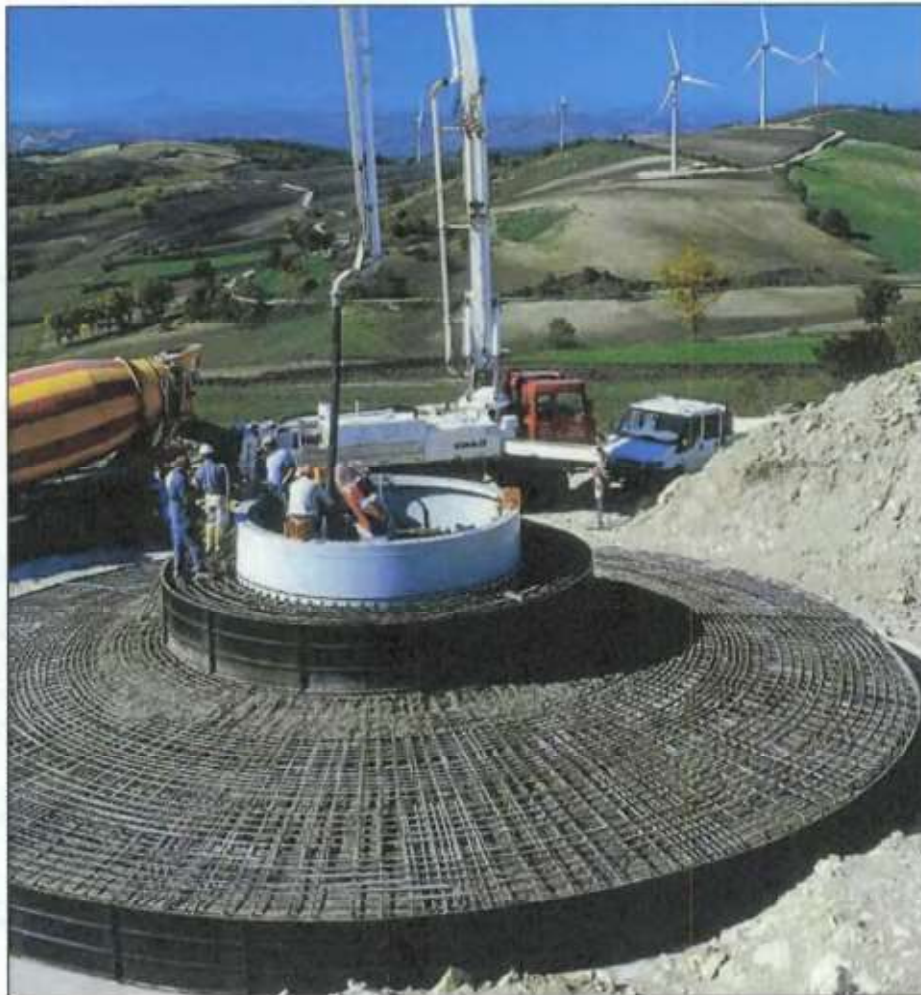
Plate 3.2: Wind Turbine Foundation 6
