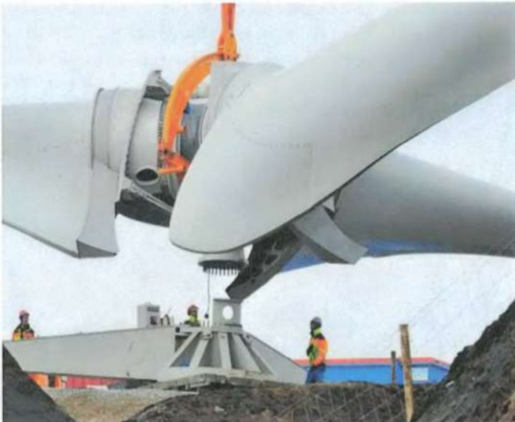
Plate 3.4: Assembly of Wind Turbine Blades 7
